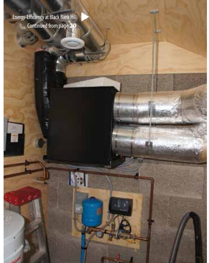
▲ Located near the pantry, the mechanical room houses an energy recovery ventilator which exhausts hot, stale air from the air-tight house and supplies cool, fresh air. While making this exchange, heat and moisture from the stale air is transferred to the fresh air, reducing energy waste with a 95 per cent heat recovery rate.
